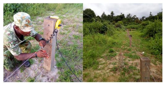
Figure 10. Electric fences to keep elephants out of fields.
